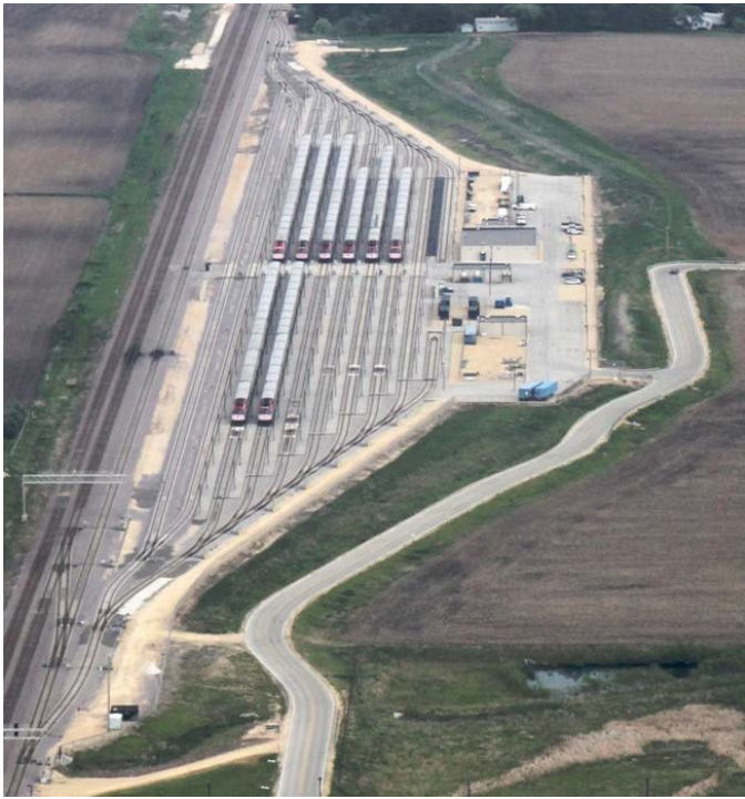
Metra Storage Yard Tracks, Elburn, IL
