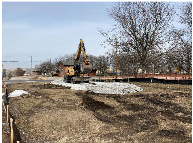
Excavation activities for utility relocations.
